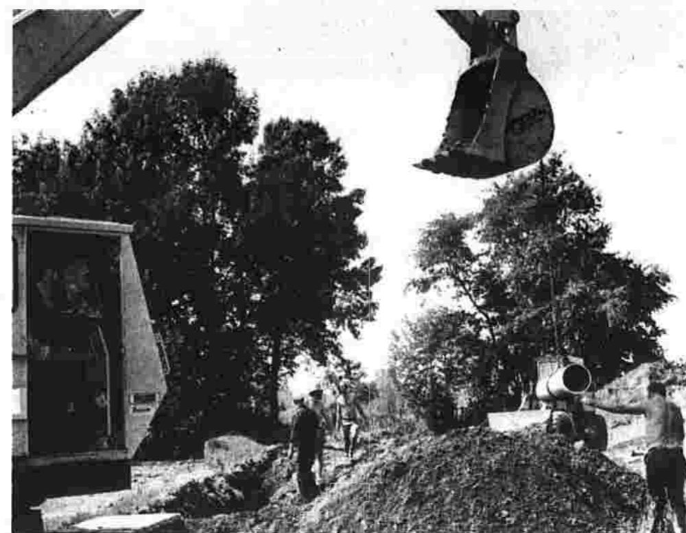
Workers install Keeney St. sewer line
