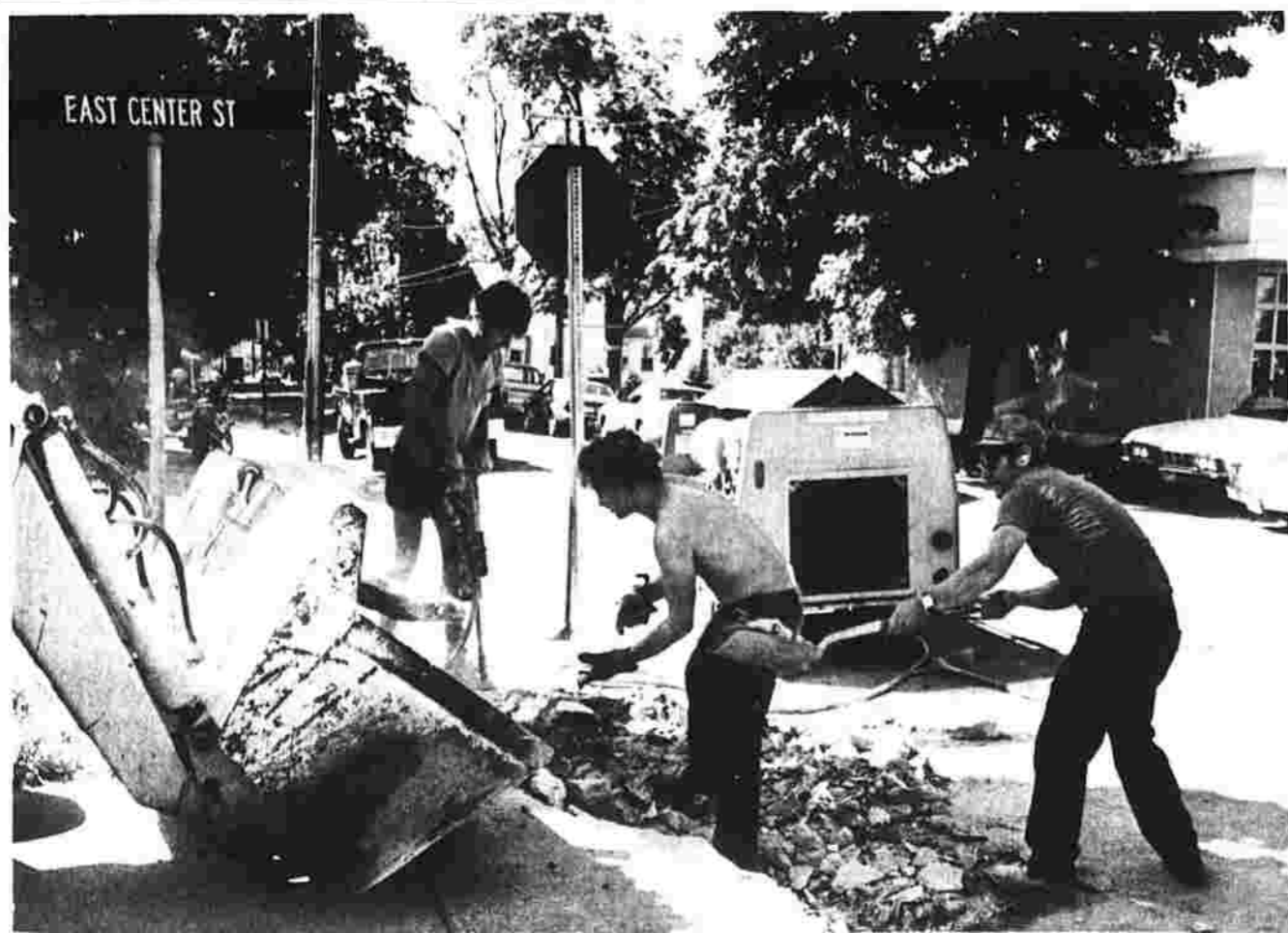
Work continues installing curb ramps
